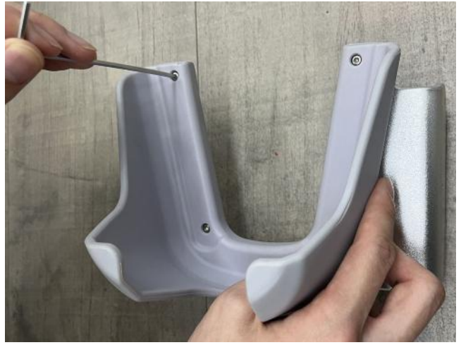
Step 7: Put the screws in the holes shown and tighten them with a hex screwdriver.
