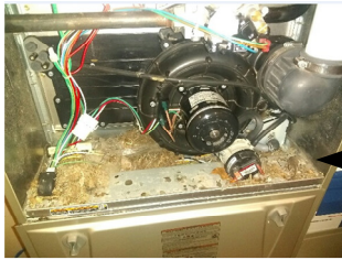
Mice in furnace from a Concentric Vent
