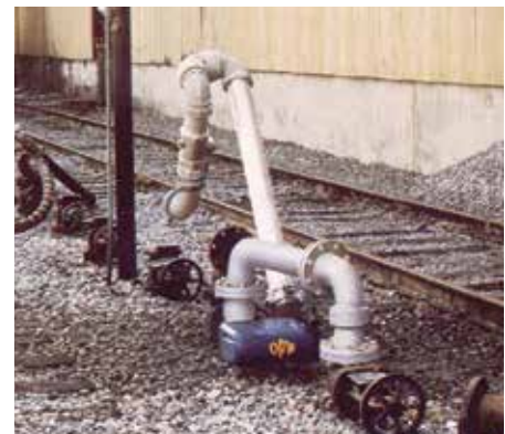
Bottom Loading Assembly
