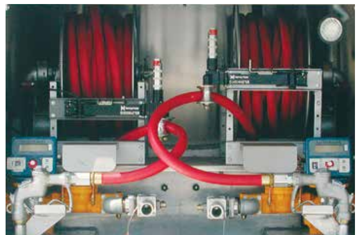
Double GuideMaster Installation
