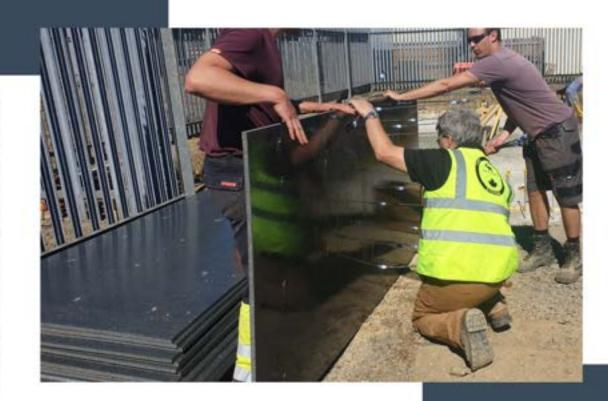
"We have now completed the solar PV project. The sheets worked very well. There are 29 solar panels on the roof with EKOply sheets supporting a weight of over 4.5 tonnes of ballast blocks. We will certainly use these again!" Chris Eades - Craven Energies
