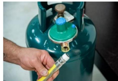
**3.** Connect the flexible hose to the pressure regulator.
