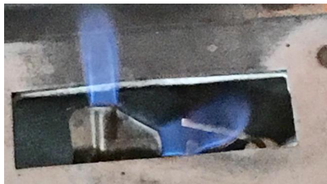
CORRECT APPEARANCE OF PILOT FLAME BOTH ELECTRODE TIP AND THERMOCOUPLE TIP IN BLUE FLAME
