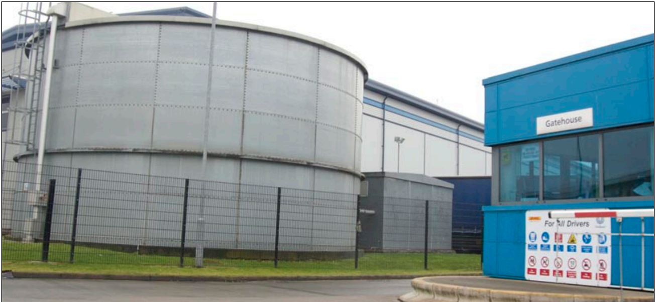
Figure 42 A firewater tank
