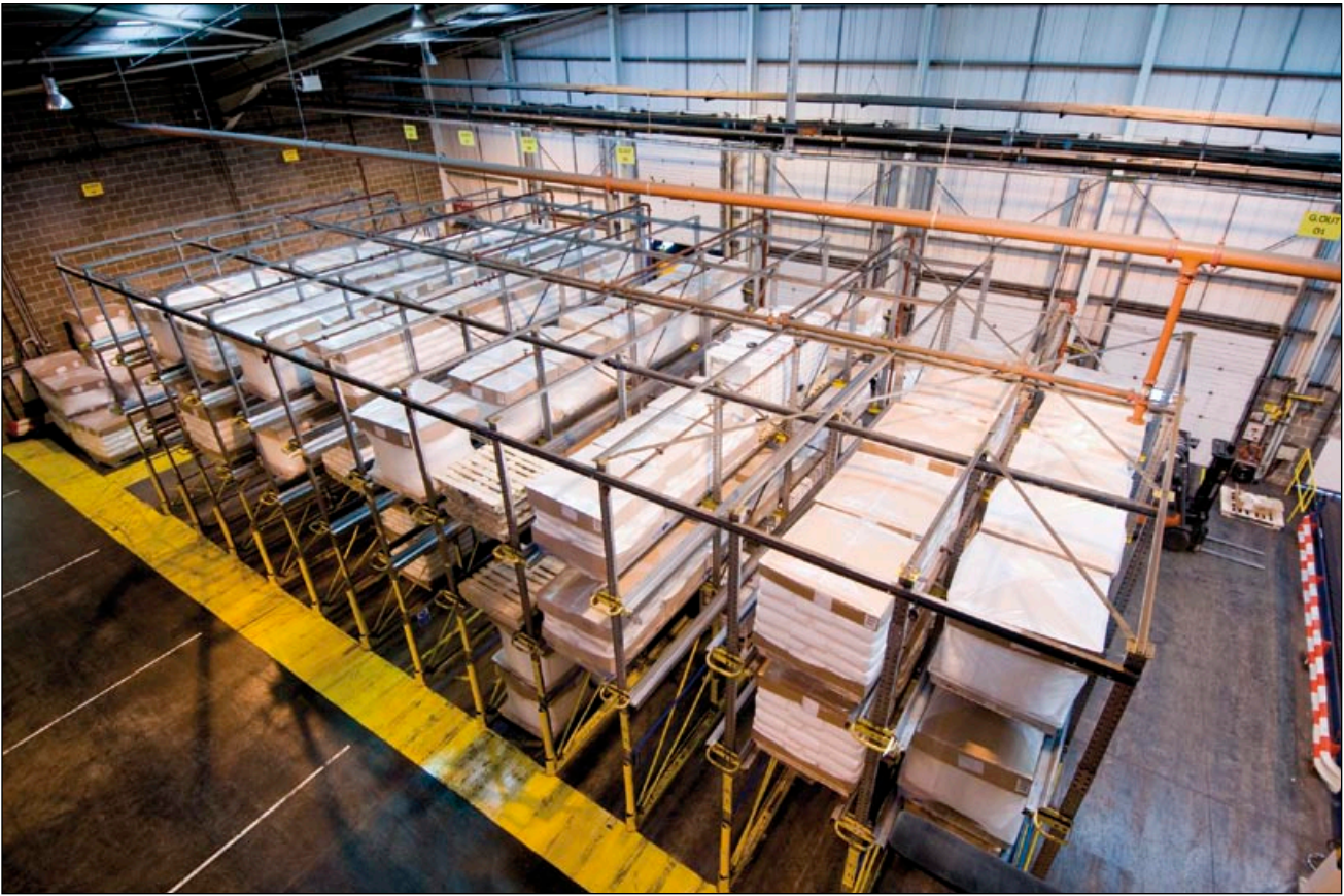
Figure 15 Storage of packaged dangerous goods in racking
