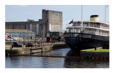
Specifically designed for long term deployment a permanent boom provided the solution to keeping the berth clean and tidy and due to the dimensions of the dock, we altered the section lengths to 10 meters to make handling easier and used a draft (material below the waterline) of 300mm and a freeboard (material above the waterline) of 150mm to suit the water state in the location.
