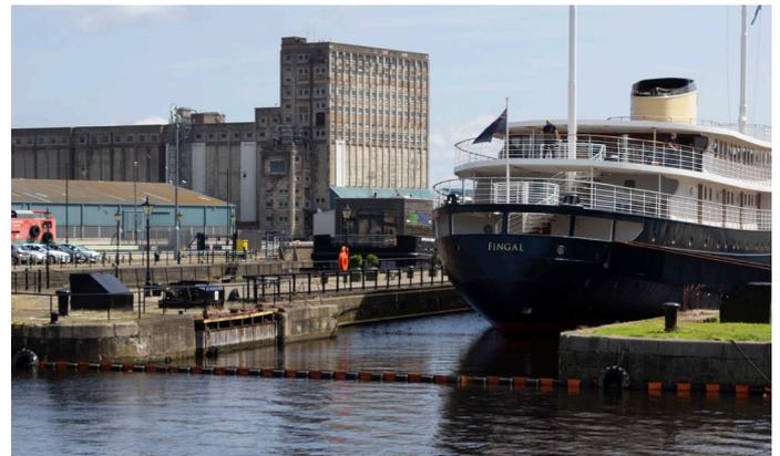
Specifically designed for long term deployment a permanent boom provided the solution to keeping the berth clean and tidy and due to the dimensions of the dock, we altered the section lengths to 10 meters to make handling easier and used a draft (material below the waterline) of 300mm and a freeboard (material above the waterline) of 150mm to suit the water state in the location.
