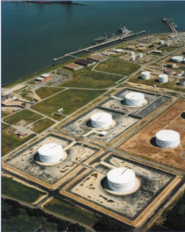
Figure 6.3 A compartmentalised bund (courtesy Seaman Corporation)
