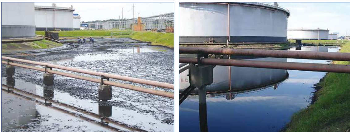
Figure 8.1 Large earth embankment bund (in service) (courtesy Oil Spill Solutions Ltd)
