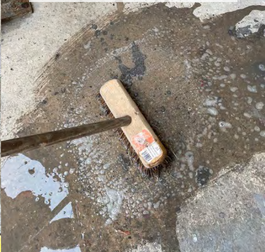
IMAGE 2: CLEAN WATER WASH DOWN
