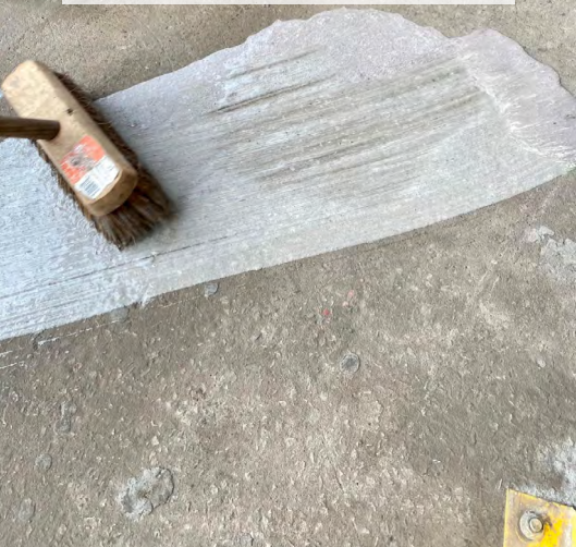
IMAGE 1: ACIDE ETCH REACTING WITH CONCRETE SURFACE
