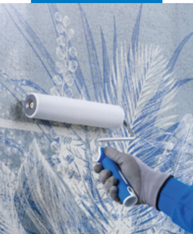
Mapecoat Decor Protection application onto decorative fiber glass
