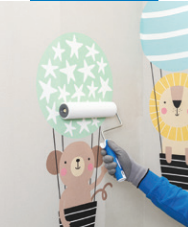
Mapecoat Decor Protection application onto printed wallpaper
