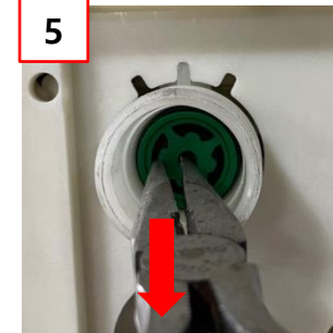
⑤ Use tool to remove the water pressure regulating valve(Green) by pulling it out
