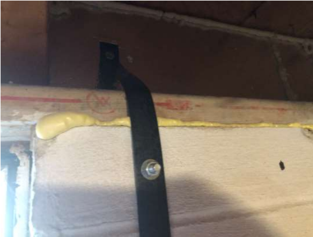
Figure 4 – Top of strap secured to sill
