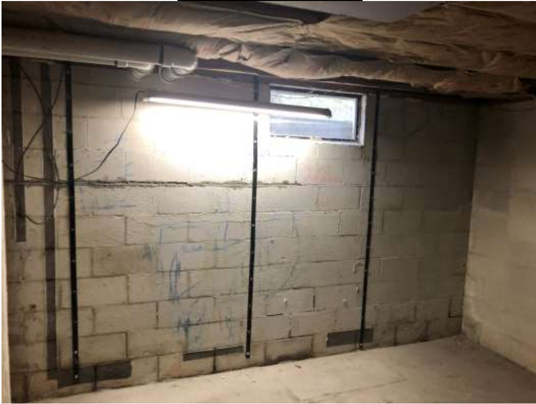
Figure 2 – Sample of installed strap
