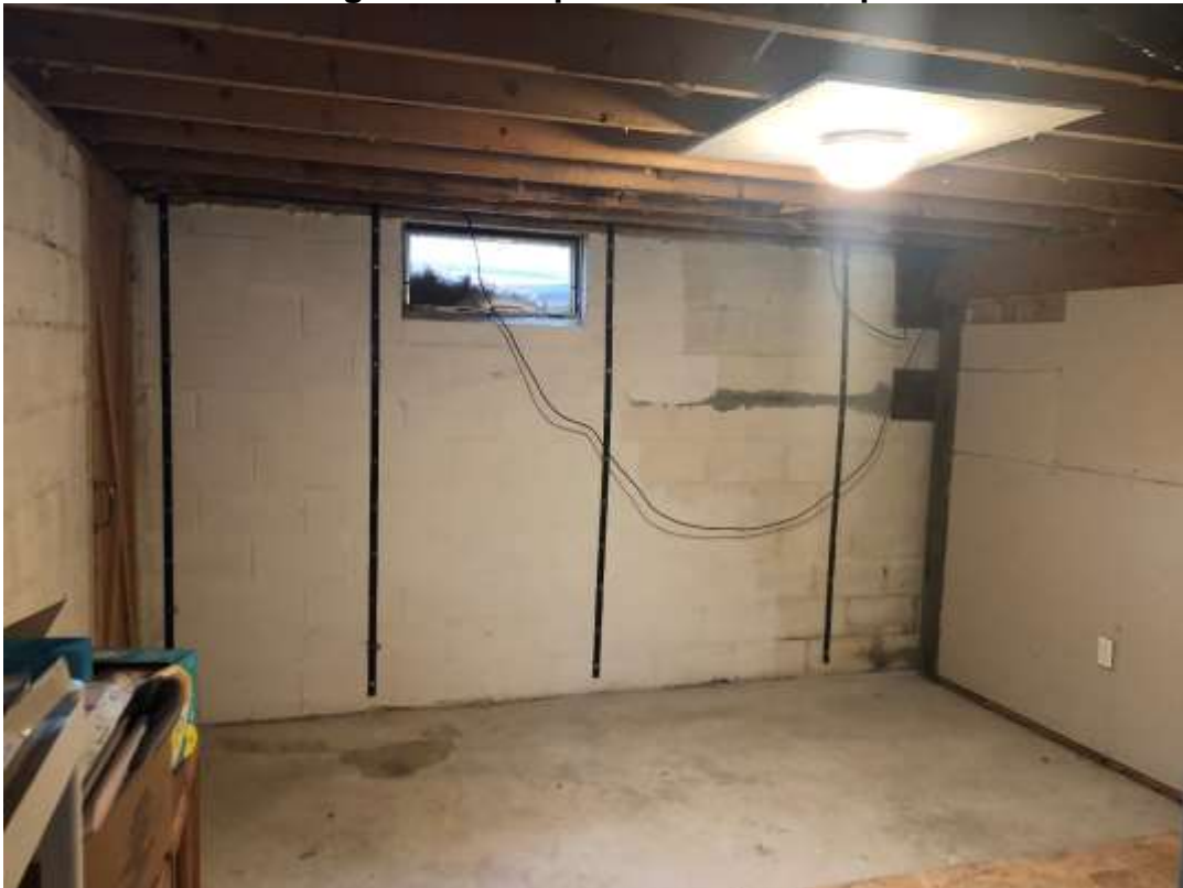
Figure 2 – Sample of installed strap
