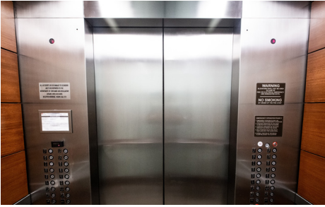
Elevator Small Room
