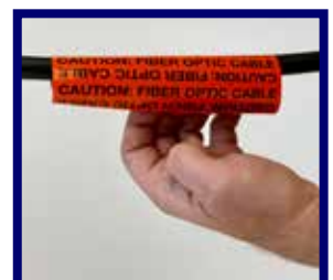
2 • Wrap around the cable.
