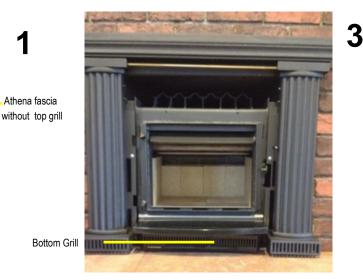
4. Fit the bottom grill on to the 2 locating screws.
