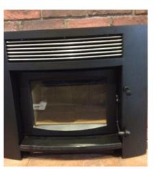
3. Place the Diva fascia against the backplate guiding the extension to the air control rod into the 'boss' (4) (the control rod hole in the fascia).
