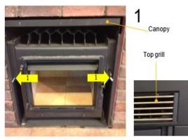
1. Remove all items from packaging and separate by releasing the bottom grill screws Remove door. Then remove the two 50mm screws (1) located one on each side of the door opening.
