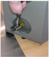
Knock the pre-lasercut opening for the aluminium hose cut with a hammer (Casing and stove body).
