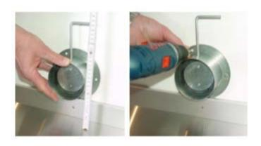
Fix the connecting piece to the wall using the screws and raw plugs provided.
