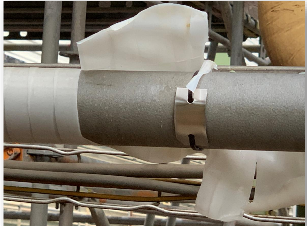
Protected Coupon After 6 Months
