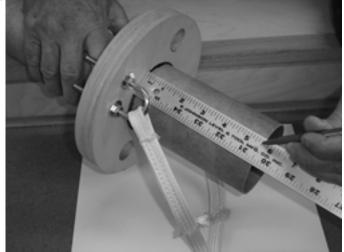
ALLOW THIS JOINT TO CURE WTH NO EPOXY RUNS ANYWHERE! Place a small drop of epoxy on the exposed u-bolt threads. Stand tube on end, Slimline end up, and allow to cure.
