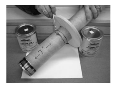
Mix a sufficient amount of adhesive epoxy and apply to the area of the tube just scuffed, within your previously made lines. Apply evenly around the circumference and slide the single centering ring back into the area of epoxy BETWEEN THE TWO PREVIOUSLY MADE LINES. BE CERTAIN THIS CENTERING RING IS "SQUARE" TO THE MOTOR TUBE AND USE TAPE TO HOLD IN POSITION.
