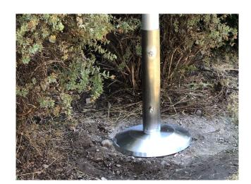
Insert the flagpole into the ground adapter and tighten side bolts.
