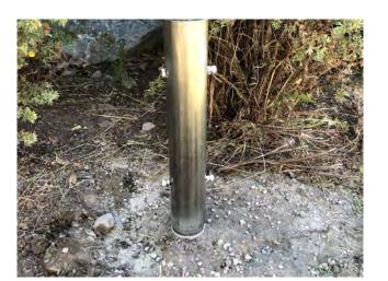
Slide the smaller end of the adapter into the existing ground sleeve.
