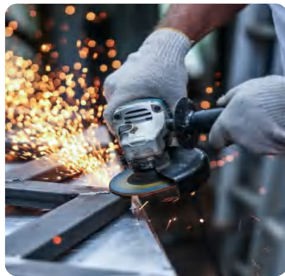
For Construction Projects
