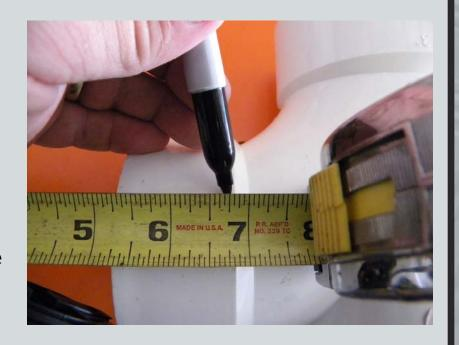
**NOTE:** Due to the difference between fitting manufacturers each assembly will need to be cut to fit.
