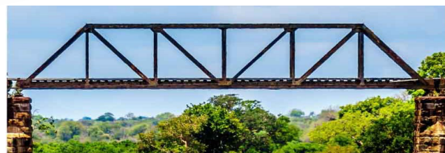
This bridge is stabilized with diagonals.
