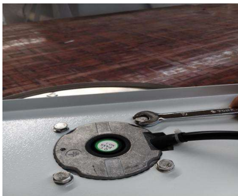
Figure 17 Dismantlement of Fan
