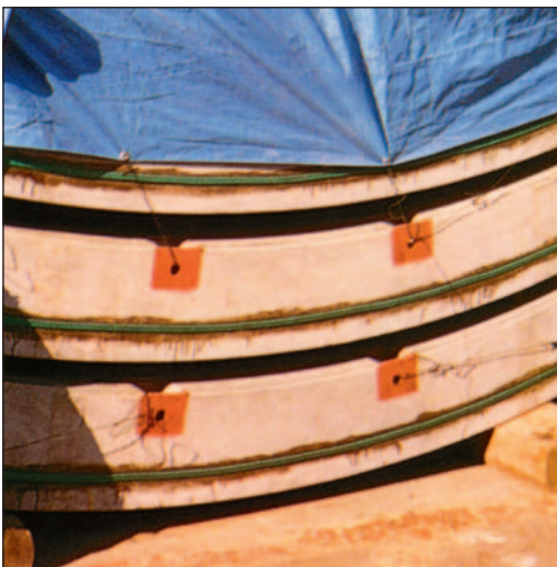
Seals between precast members
