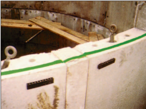
Seals horizontal and vertical cold joints
