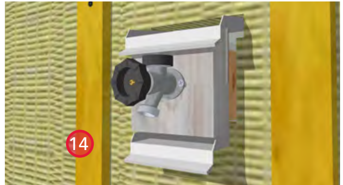
14. Install the bottom block and sill flashing. The sill flashing is fastened to the back of the bottom block.
