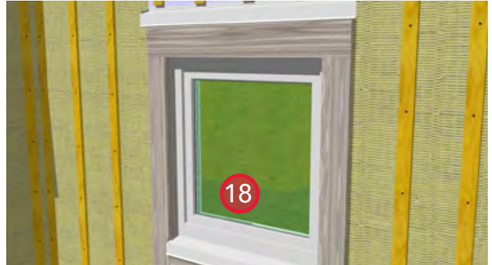
18. Install window trim boards.
