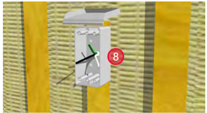
8. Install electrical box.
