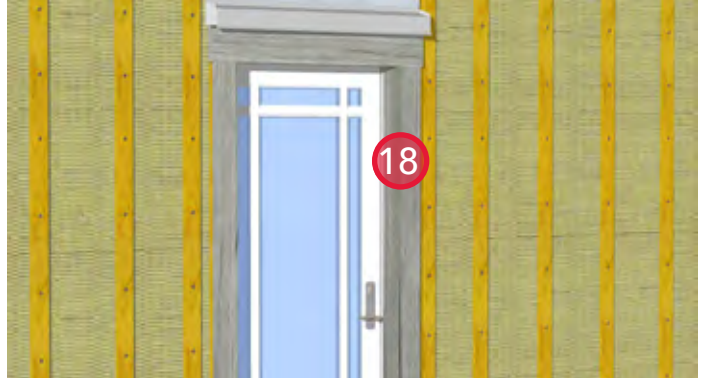
18. Install swing door trim boards.
