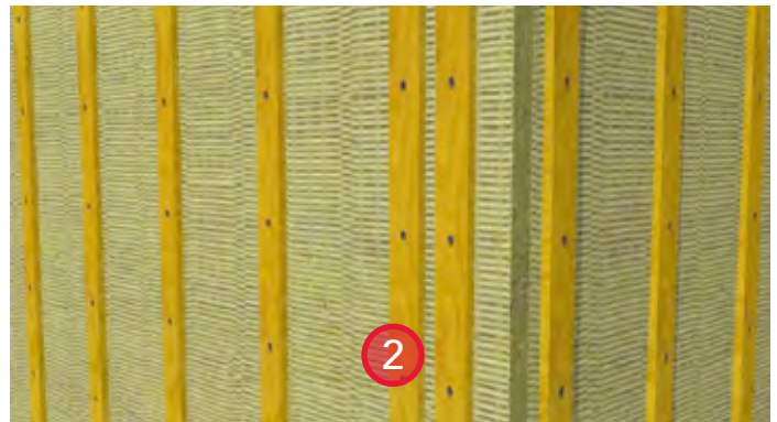
2. Install ROCKWOOL COMFORTBOARD™ 80. Use the strapping to support the insulation and secure in place with recommended fasteners. Provide bugscreens at the top and bottom of the strapping.
