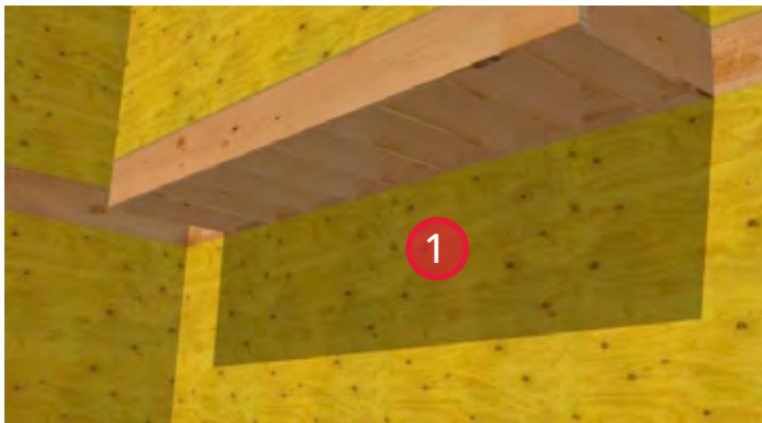
1. Typical wood frame construction at sheathing stage.
