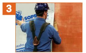
Gradually peel off the remaining silicone release paper, making sure the membrane adheres completely to avoid air pockets and wrinkles.
