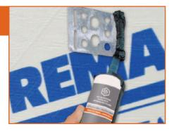
Use SOPRASEAL SEALANT to seal around details, reverse laps, critical areas and window openings.
