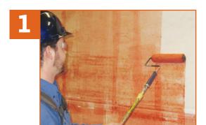
Prime the substrate with SOPRASEAL STICK PRIMER, ELASTOCOL STICK ZERO or ELASTOCOL STICK  $H_2O$ .
