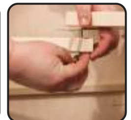
Replace wood brace and wing nut
