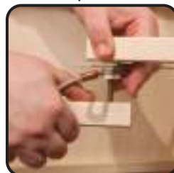
Remove wood brace
