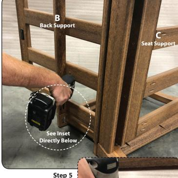
Turn the entire assembly on its side. Keeping the back support (B) flush with the armrest-leg assembly (A), fasten the back support to arm rest with (2) 1 1/4" screws through holes in back support, see inset picture on right.
