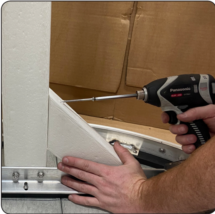
Step 4 Then attach the same brace to the leg with (1) 2" screw, as shown.
