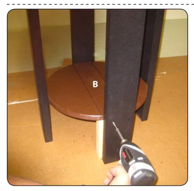
**Step 2**Turn table upright. Now fasten shelf using (8) 2 1/2" screws. Align screws with pre-drilled holes in shelf.
