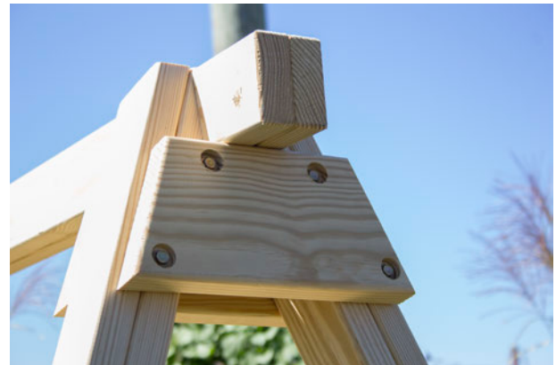
Top Brace connection shown
