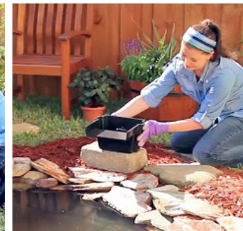
2. Place the spillway based on your measurements
