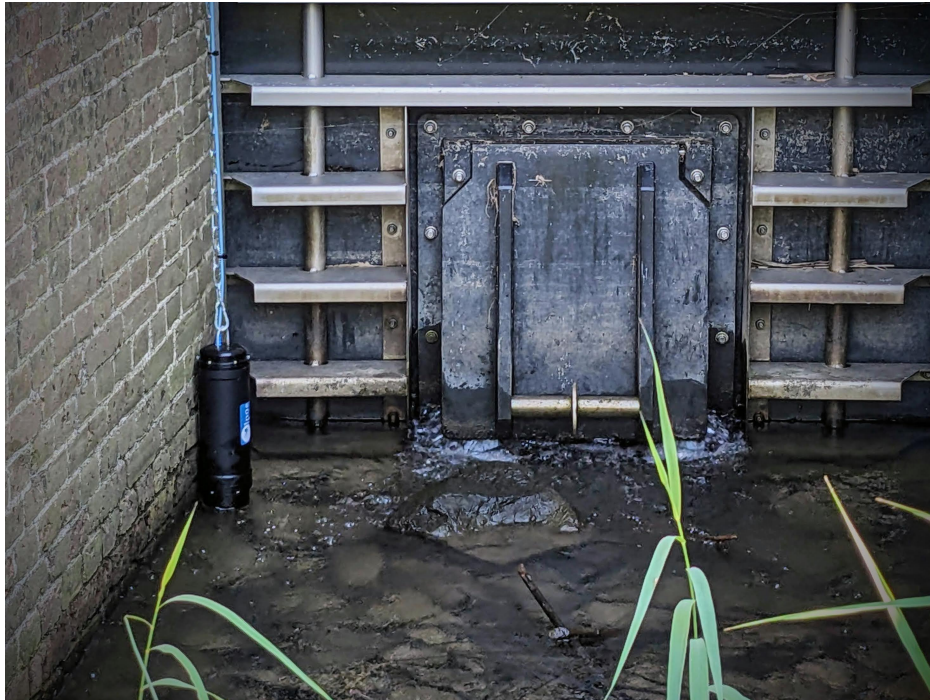
Figure 4. Olpas sensor (v1) installed in an overflow at nature side.
