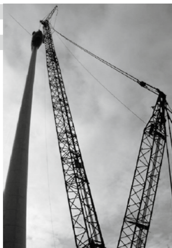
LARGE LATTICE MOBILE CRANE (Enercon E82 on 98 m tower)
