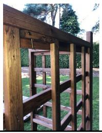
Insert 4x 35mm screws in the pre-drilled holes down each side of the trellis and fix from the back through the support bars into the trellis.
