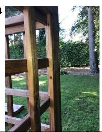
Position the back trellis between the two sides. Fix in place with 2x 50mm screws through the top support block.
