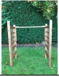
Fix top support bar in place with 2x 50mm screw on each end of the bar.
