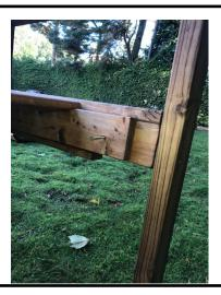
Fix in position using 8x 70mm screws 4 on each side evenly spaced.
