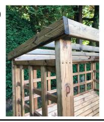
Position the roof frame on the arbour, ensure it is flush to the back legs, lift the front of the roof so it is flush with the top of the front legs and fix in place with 8 100mm screws. Pull the canvas sunshade over the roof frame, remember to remove the canvas sunshade during inclement weather.
