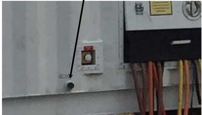
External fuel drain fitting.
