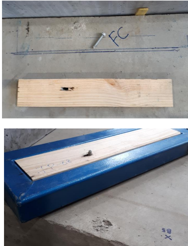
Figure 14: Anchor in shear failure
