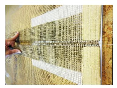
• Finally fold inside the thread to secure the closure.
