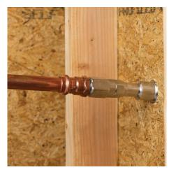
2) Hand tighten new inlet on hydrant body by threading clockwise.
