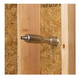
1) Remove existing inlet by unscrewing counterclockwise. Ensure the O-ring on the hydrant body is properly seated.
