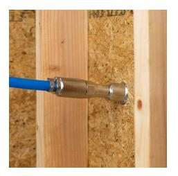
3) Attach to PEX tubing using appropriate tool and clamp or crimp ring. Check for leaks and test the hydrant operation.
