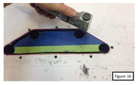
21. Trim or grind excess hood material away until the hole in the hood matches the template, and the center hood vent will drop into the hole with a little bit of wiggle room.
