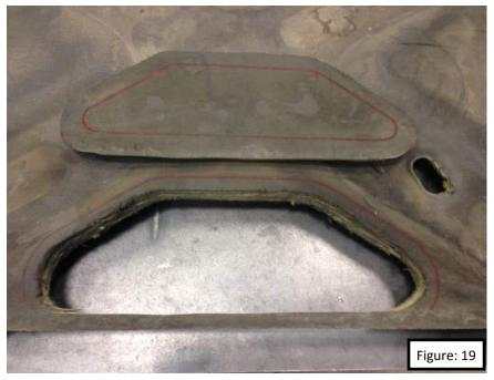
34. Make sure the cut out in the heat hood blanket is large enough for the vent ring to fit with a little wiggle room.
