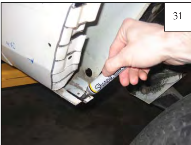
Mark cut lines on exposed sheet metal
