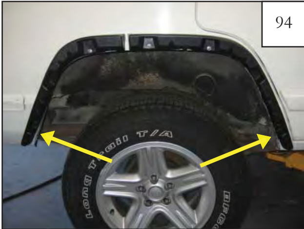
Install tuflocks in two lowest hole locations on inner pieces P3 & P4 (D3 & D4 for driver's side).
