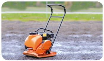
Run your compactor over the grid, making sure to **compact all areas including the edges**. If compaction is lowering the gravel enough that the grid is exposed, add some more gravel to the affected cells.
