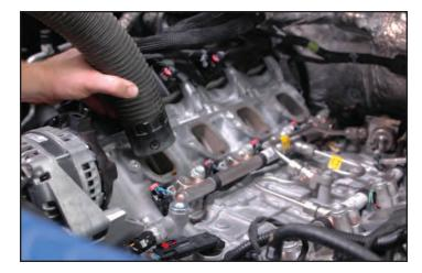
30. Use denatured alcohol, lacquer thinner or some other non-petroleum based solvent to wipe the surfaces of the head intake ports.
