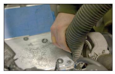
55. Remove the Steam Vent hose from the hose barb by squeezing the spring clamp to release the hose, then pull free.
