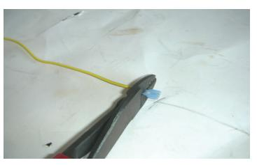
110. With the relay mounted, take the yellow trigger wire from the relay, strip about ¼" of the insulation from the end and crimp it onto the supplied spade connector.
