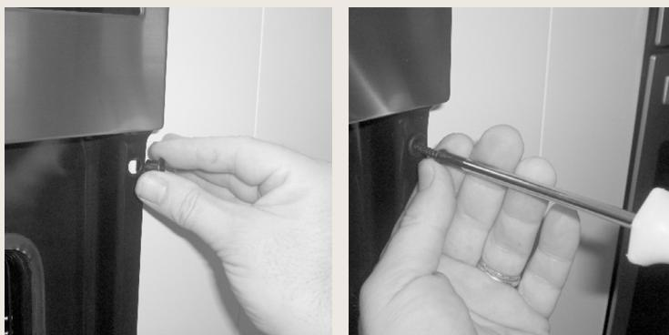
Use the four screws provided to fasten the bushings to the cabinet, taking care not to over tighten and break the bushing.
