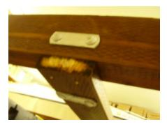
Note that the carriage bolts are installed so that the flat head is out and on the bottom side. It is safer to have the bolts installed this way to prevent possible head injuries to a person should they swim under the dock.
